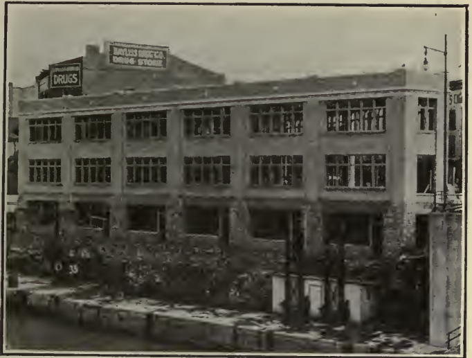
WHERE WAS FORMERLY A LOCAL EYESORE THE LOCKPORT, N. Y., BOARD HAS BUILT ITSELF AN ATTRACTIVE HOME
